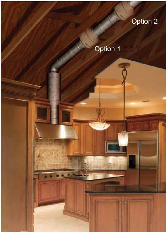
The fans can be connected at any point along the ventilation duct: along the duct or at the end.
